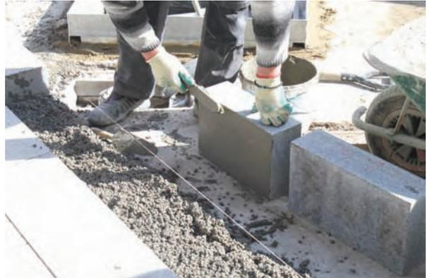
Paving units are to be beaten with the maul firmly to line and level without delay and thereafter they are not to be disturbed. The short level is frequently used to slide across the freshly laid paving units, the check for lips. The long level should be frequently used to check level over wider areas.
