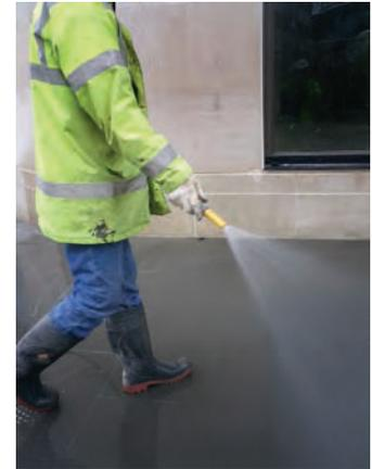
The process of wetting and removal is repeated, water always being applied to the surface in the form of a fine spray, taking care not to disturb the mortar in the joints. The surface is thereafter maintained in a damp condition by periodic application of water in the form of a fine spray. It should never be allowed to dry, even in small places, until final cleaning is effected.
