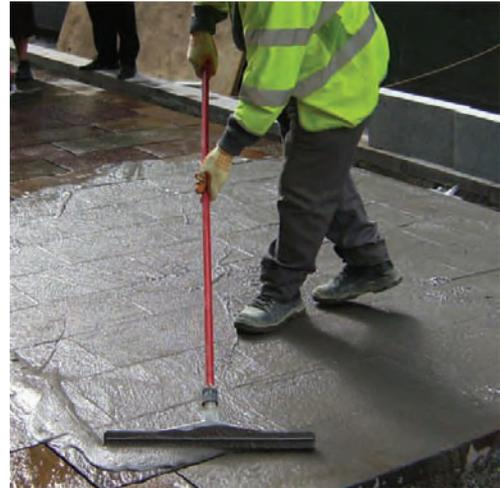
Fresh mortar is allowed to settle within the joints and fresh mortar is drawn across the surface repeatedly until joints are full and further settlement has ceased.
