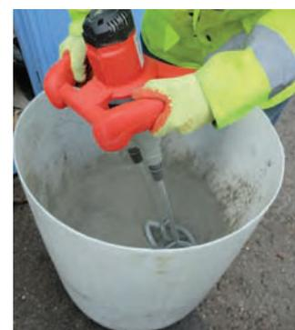
Mixing should be made using a powered paddle mixer, either hand-held or stationary. Manual mixing is not good practice due to the risk of incomplete blending.
