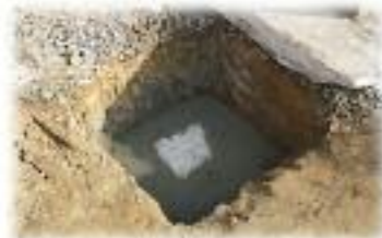
2 Excavate for pump chamber
