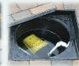
8 Connect pump and system ready for use.
