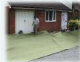
5 Lay Inbitex Geotextile
