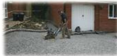
4 Spread and compact 5-20mm clean stone
