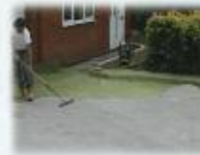
6 Spread and screed 2-6mm clean stone
